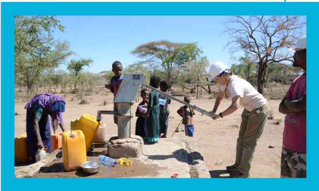
Afar, Ethiopia: A professional volunteer from Engineers Without Borders USA's Engineering Services Corps repairs a hand pump to restore water to a drought-stricken community. (Photo credit: Erin Cummings)
